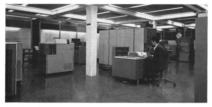
Brokers who subscribe to the SCAN system operated by Intinco Ltd. of London can get immediate, up-to-the-minute data on stocks and shares and instant answers to enquiries through a small keyboard in their own offices. Intinco's UNIVAC 418 Real-Time system works both ways. So brokers can hold a keyboard "conversation" with the computer.
