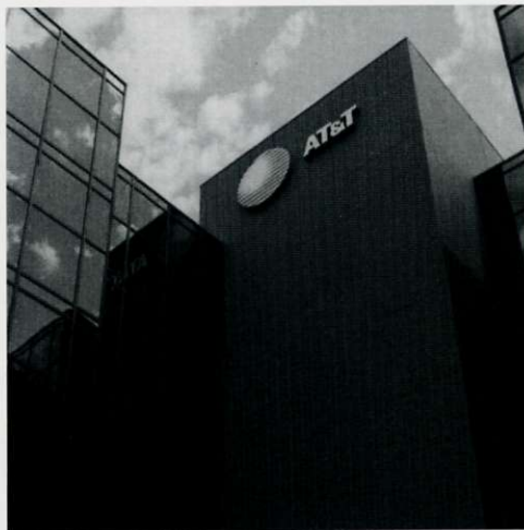
AT&T GIS World Headquarters building in Dayton, Ohio.
