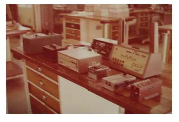
The next two pictures show the Board Comparator Tester I built. This tester compared a good and bad board. A plug-in patch board was used to program the board under test. The patch boards simply identified to the Tester which pins were Input pins and which pins were Output pins. The Tester, when run, applied a binary sequence (to cover all possible combinations) pulse to all the
