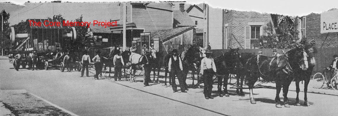
Part of the Corliss on its way to the NCR power house in 1902. Five teams were required to move it.
