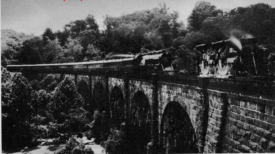
The Thomas Viaduct on the B & O between Baltimore and Washington spanning the Patapsco River is the oldest railroad stone viaduct in the world. Built in 1835, many said it would not even support the three-and-a-half-ton Grasshoppers. Yet it has never faltered under the heaviest of modern trains.
