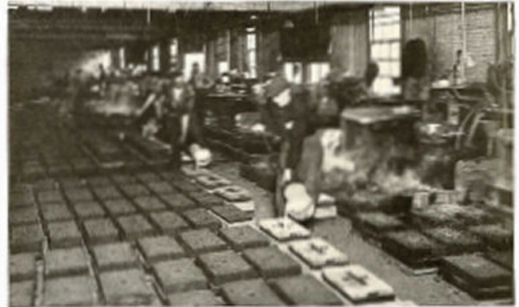
The castings used in building our product are made in our own foundries
